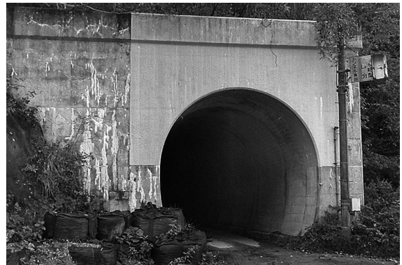
Fig. 1 Appearance of Yunose Tunnel.
